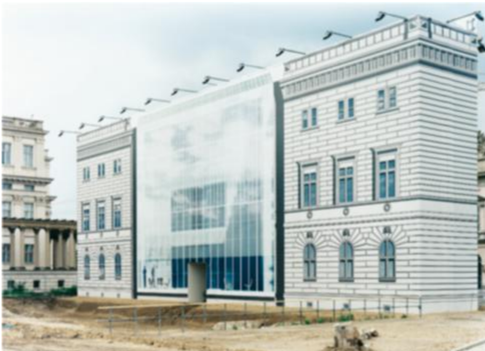
Digital simulation mounted on scaffolding. Bertelsmann Media Group bought the land with the prestigious address Unter den Linden 1 to build a new representative headquarter in the German capital. The building is a mix of the reconstruction of Berlin's former Stadtkommandantur or city garrison headquarters, which stood on that land historically, but did not survive WWII. This is the modern rear view. During Bertelsmann's annual summer event, a huge party tent was erected behind the simulation. Limousines stopped in front, and guests literally walked through the simulation into the party tent.
